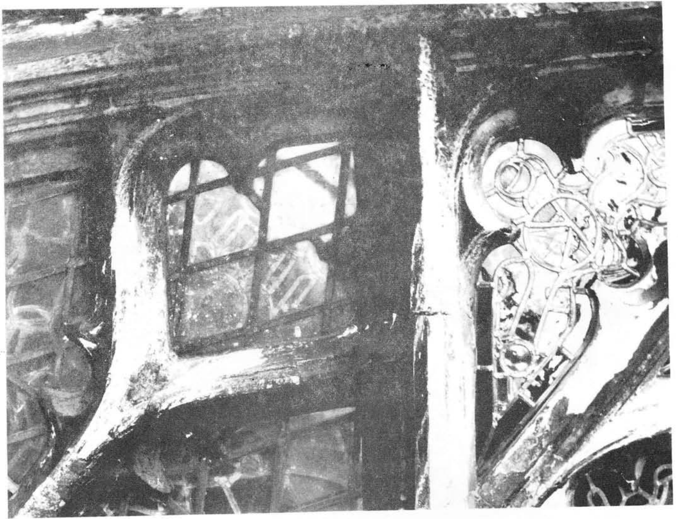
Fig. 3 The external glazing has been removed from the panel on the right.
