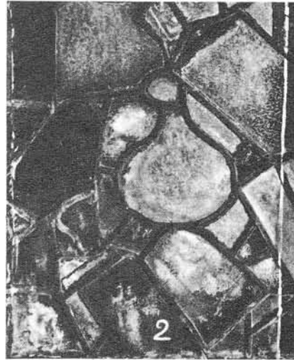
Panel No.2 at St Maria-am-Gestade, as photographed in 1976, after exposure to the atmosphere for 5 years in an unprotected state. By courtesy of Dr Bacher and the Bundesdenkmalamt, Neg. No.N71167.
